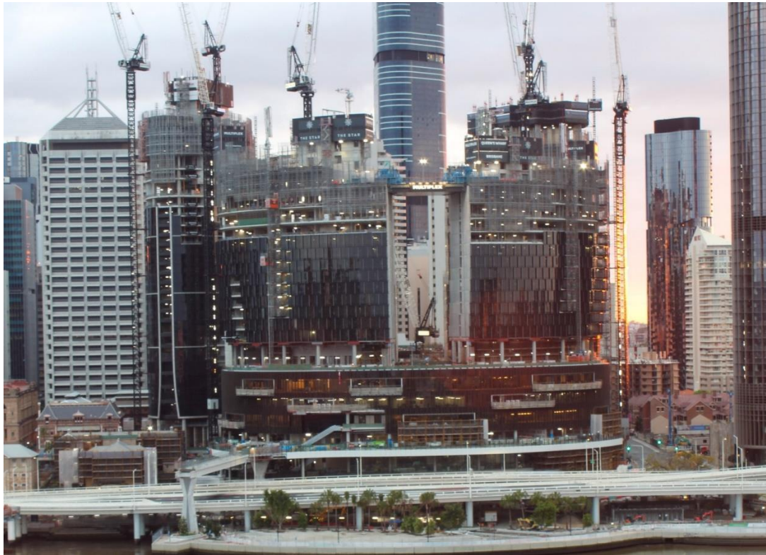
Image: Sky Deck platform in place
